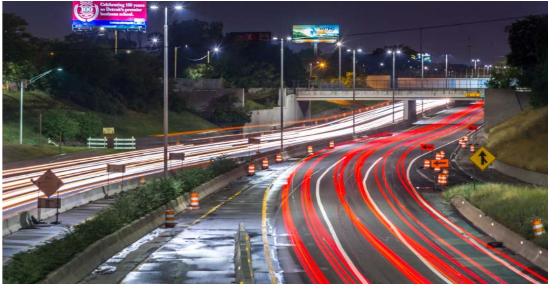
Metro Region Freeway Lighting – Availability Payments
